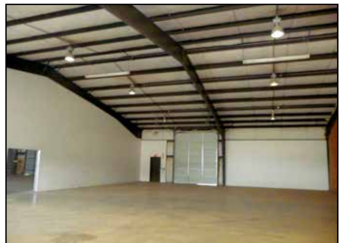
Interior bay in Building on Parcel B
