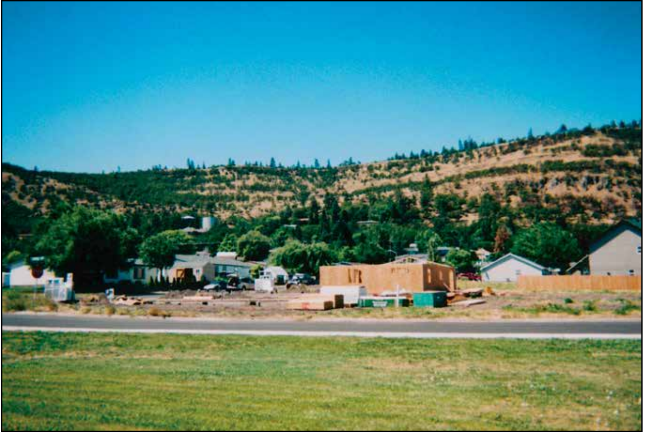
New home under construction
