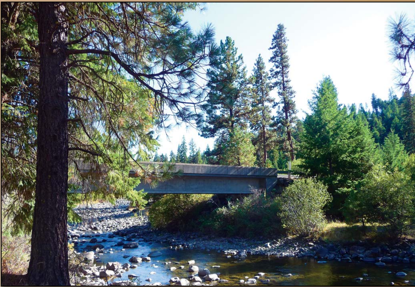
USFS Road 1003 bridge in northeast section of property
