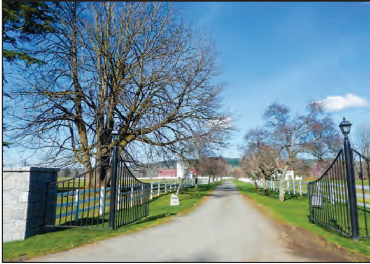
Main entry gate
