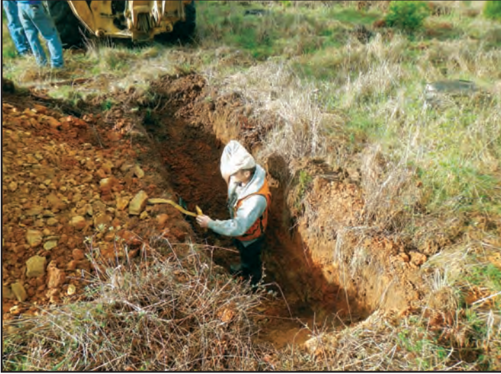
Soil test on site in 2014
