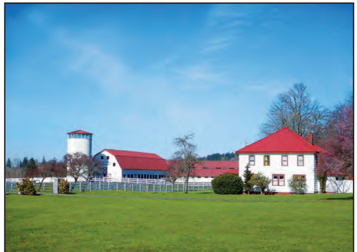
Caretaker residence and barn
