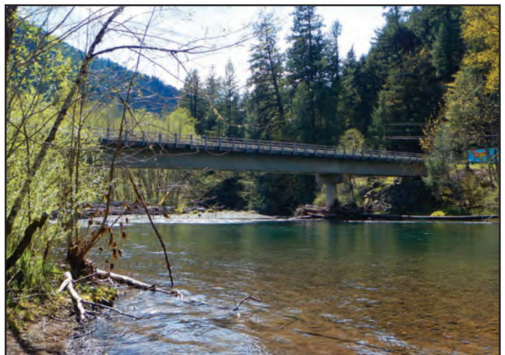
Quartz Creek USFS bridge
