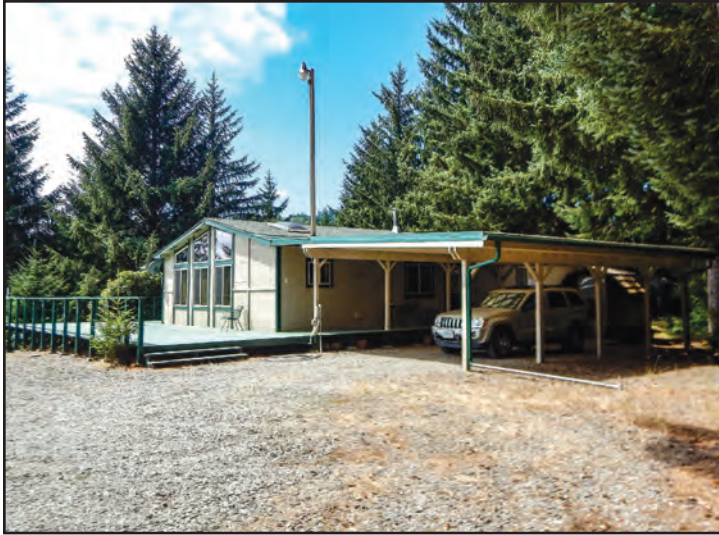
Three bedroom, two bath main residence
