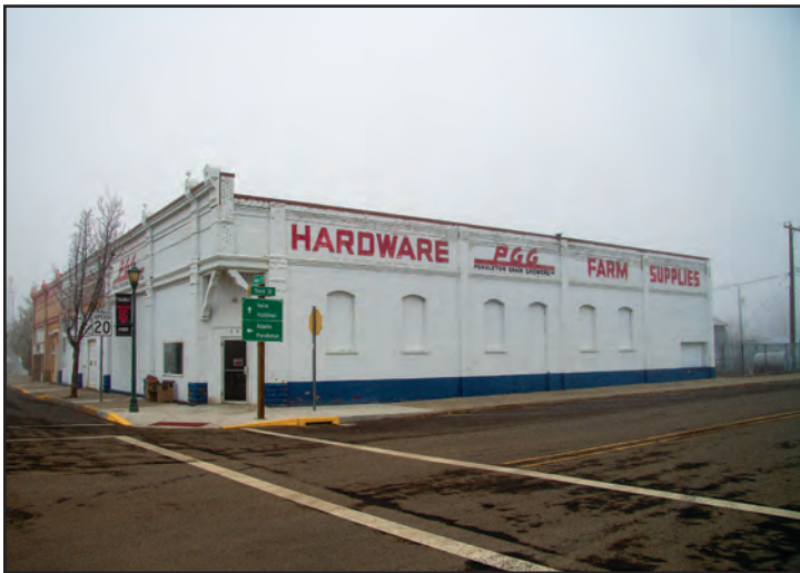
Building, and 12,000± square foot lot, have options for reuse and redevelopment
