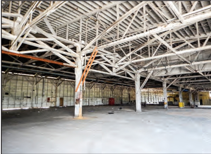
Over 100,000 square feet in main mill building
