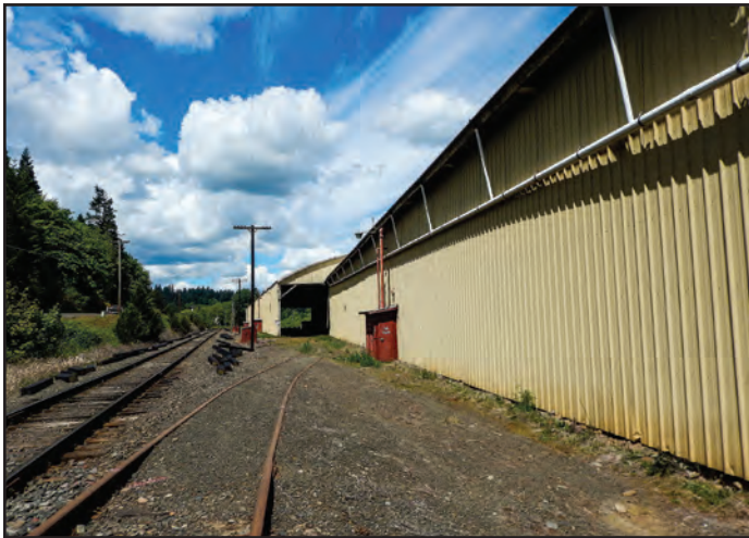
Rail spur into main mill building
