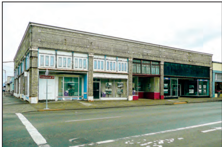
Auction Property #103: 8,125± s.f. Commercial Building in Astoria Historic District
