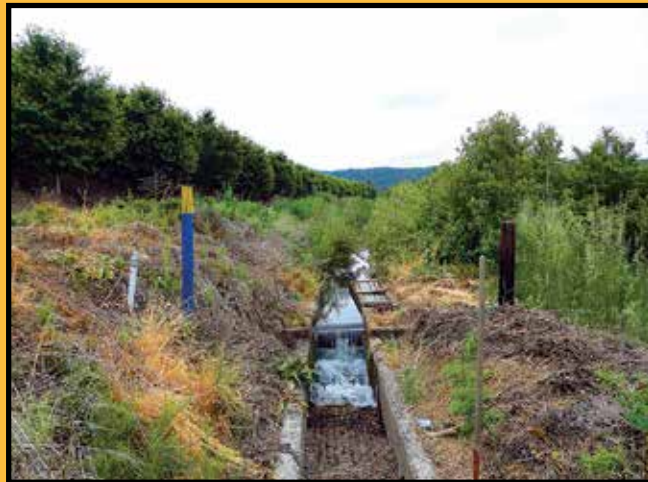
Irrigation canal in West orchard with 80% of system being gravity fed
