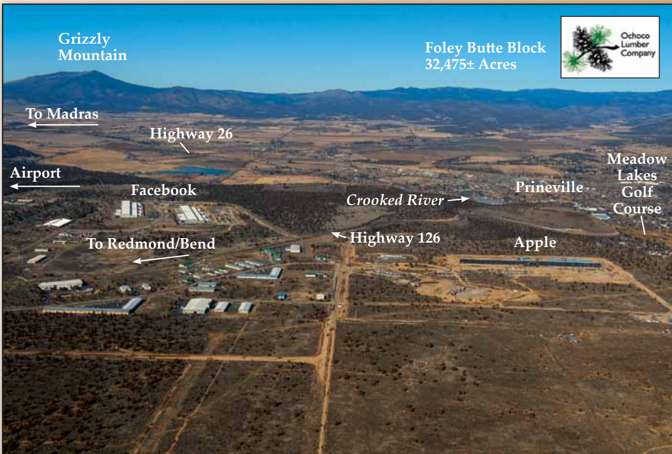
Foley Butte Block may be one of the largest contiguous blocks of private ownership near Prineville, which is home to Facebook and Apple Data Centers
